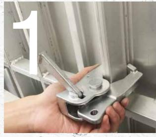
Press Fastener open to fix on the grooves of the Formwork Panels
